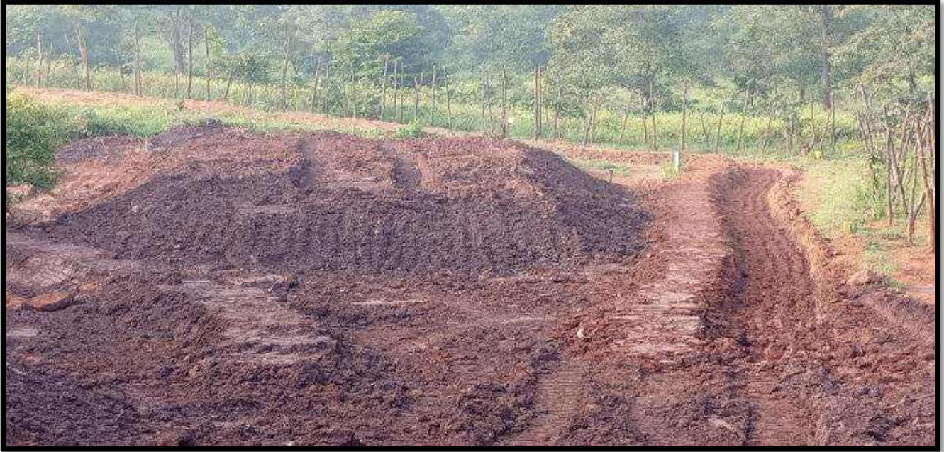
Photo-3 Generated top soil are kept at ear marked location
