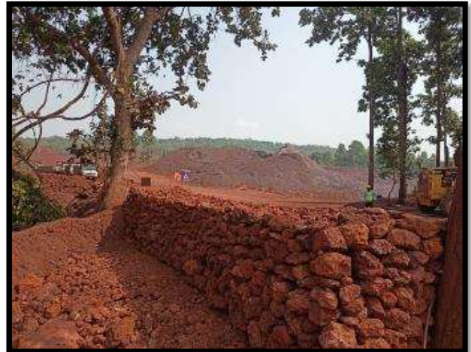
Photo-10 Settling pond with Check Dams in defferent locations
