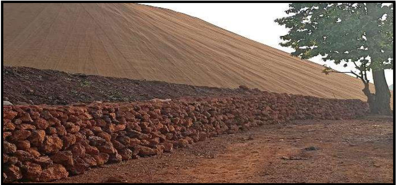
Photo # 9 Geo textile mat laying on waste dump & fines dump Slop
