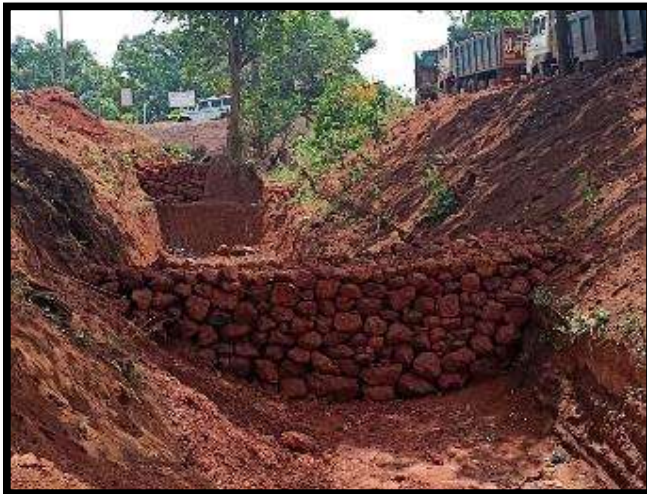
Photo-10 Settling pond with Check Dams in defferent locations
