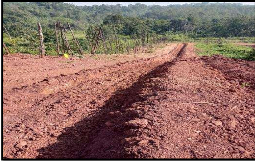
Photo-1 Showing the Garland Drain at the toe of OB Dump
